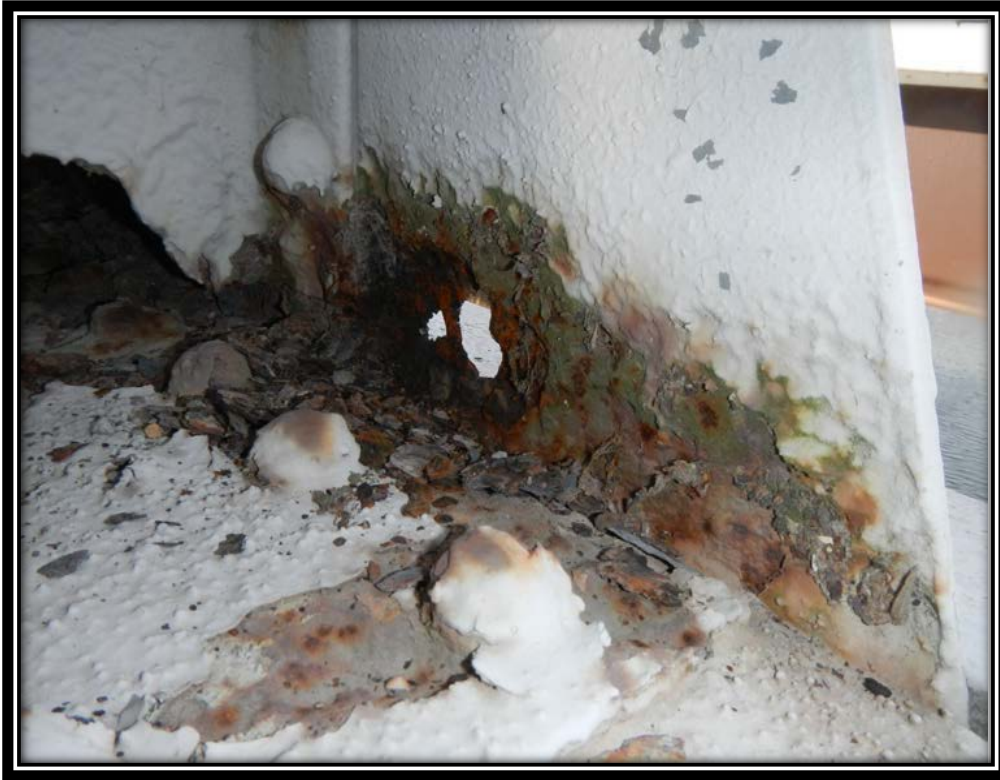
Looking northwest at the outboard gusset plate at L2, span 17, north truss. Note: 1-inch diameter corrosion hole through the gusset plate along the horizontal shear plane.
