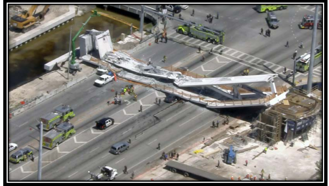
Miami bridge collapse
