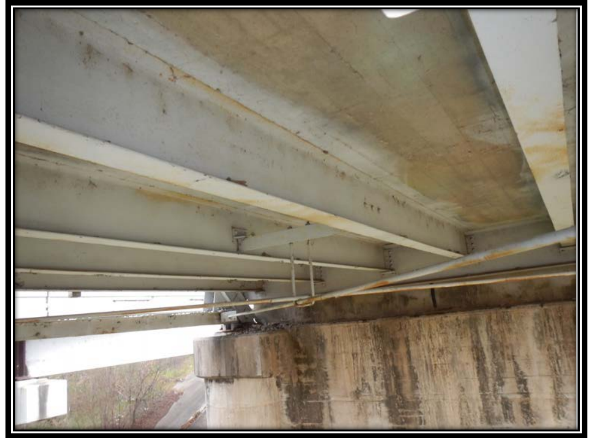
Looking northeast at the stringers at floor beam 8. Note: typical stringer condition with minor surface corrosion on the webs and flanges.
