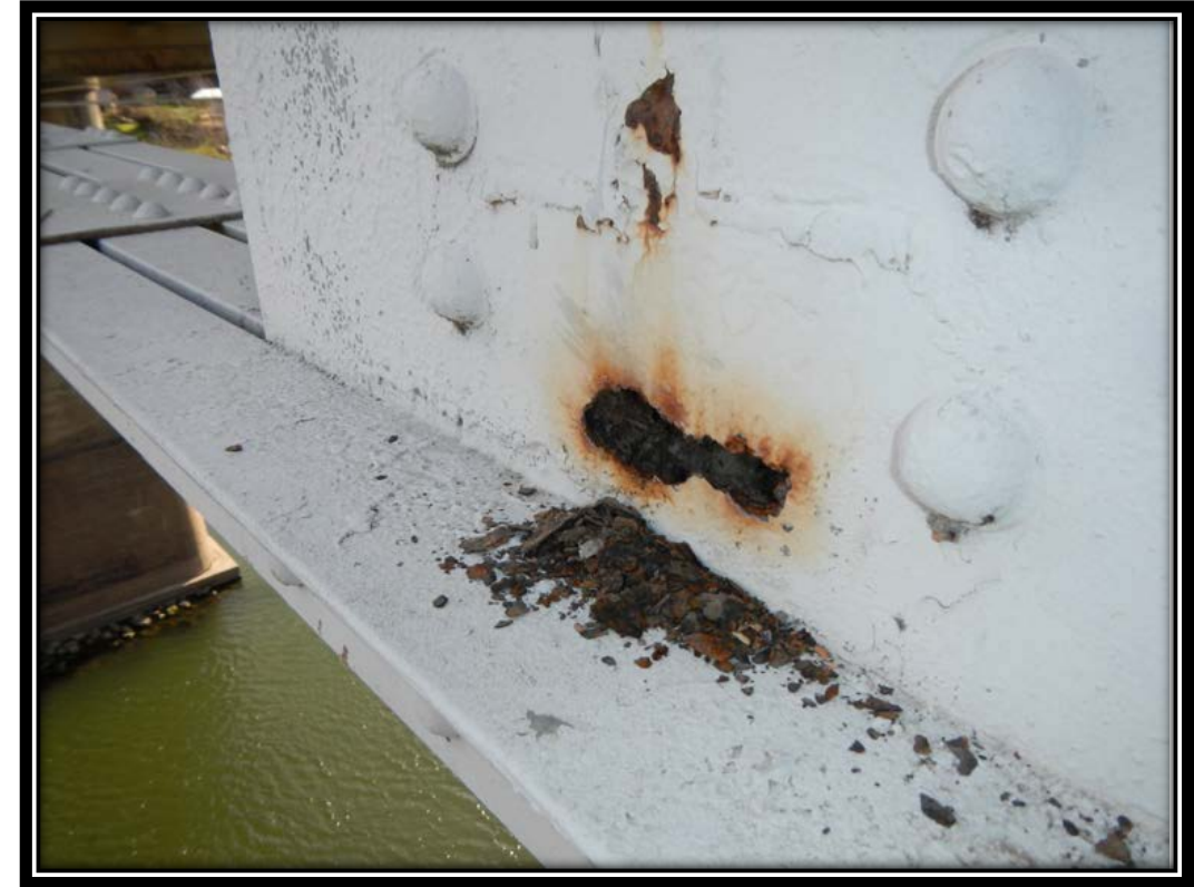
Looking southeast at the outboard gusset plate at L4, span 17, north truss. Note: 3 1/2-inch horizontal by 1-inch vertical corrosion hole through the gusset plate along the horizontal shear plane.
