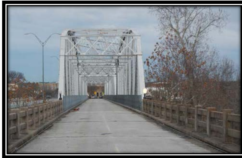
End view looking east.
