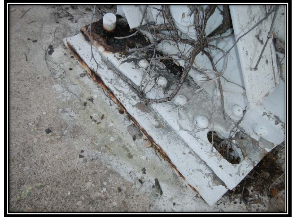
Looking southeast at the north truss bearing at L0, north truss. Note: one missing anchor bolt on outboard face of the bearing. Also note, expansion slot filled with corrosion and debris.
