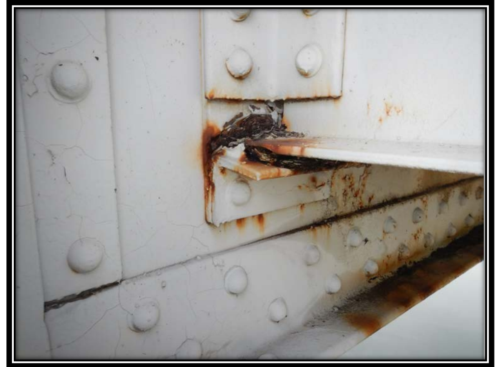
Looking northwest at stringer 6 connection to floor beam 3 in span 17. Note: heavy pack rust between stringer bottom flange and seat angle.
