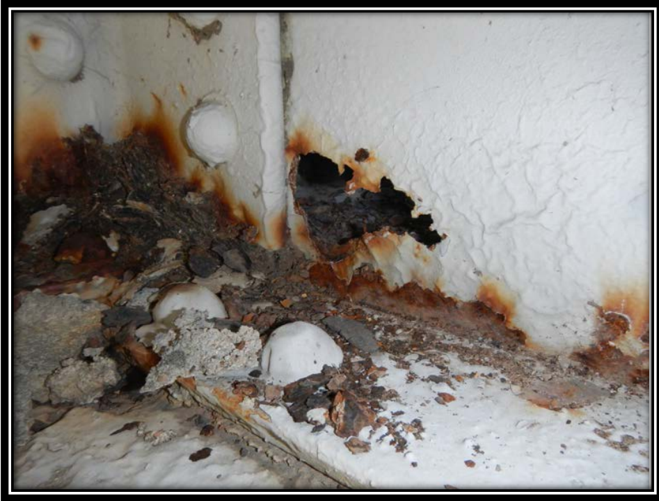
Looking northwest at the inboard gusset plate at L6, span 18, north truss. Note: 3 1/2-inch horizontal by 2 1/2-inch vertical corrosion hole through the gusset plate along the horizontal shear plane.
