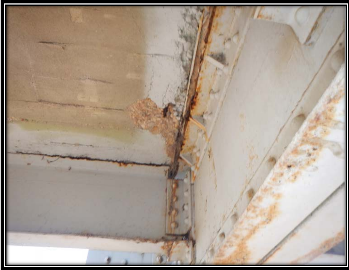
Looking north at the underside of the deck at floor beam 3 in span 16. Note: spall in deck underside with exposed reinforcing steel adjacent to floor beam top flange.
