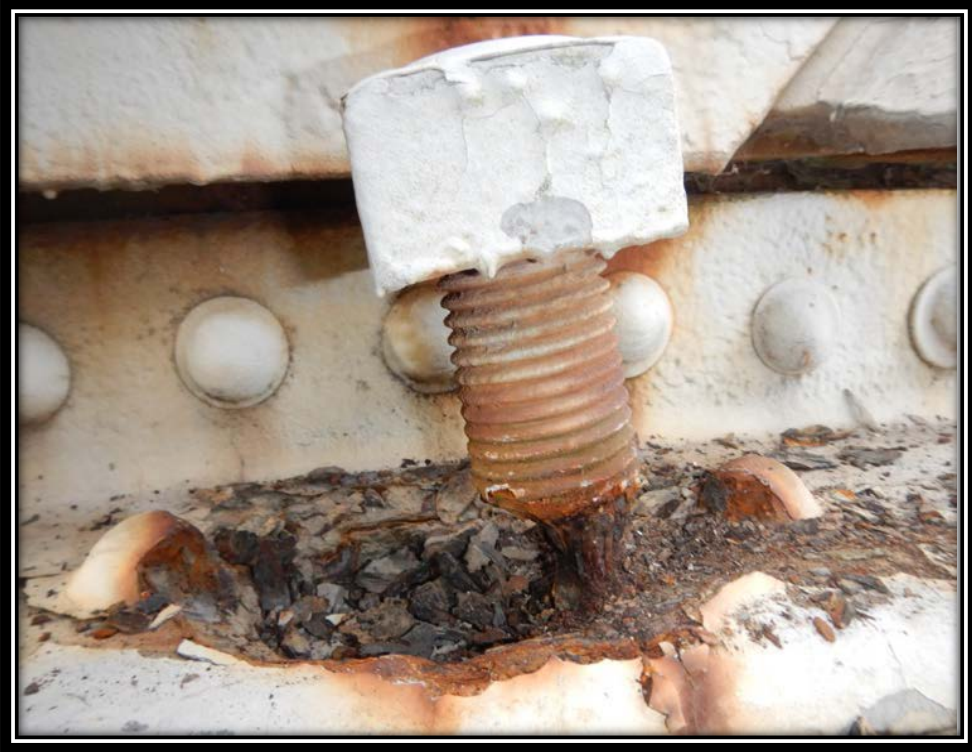
Looking north at the south truss bearing at L0, span 17. Note: 1 1/2-inch nominal diameter anchor bolt exhibits up to 75% section loss at the base of the anchor bolt.
