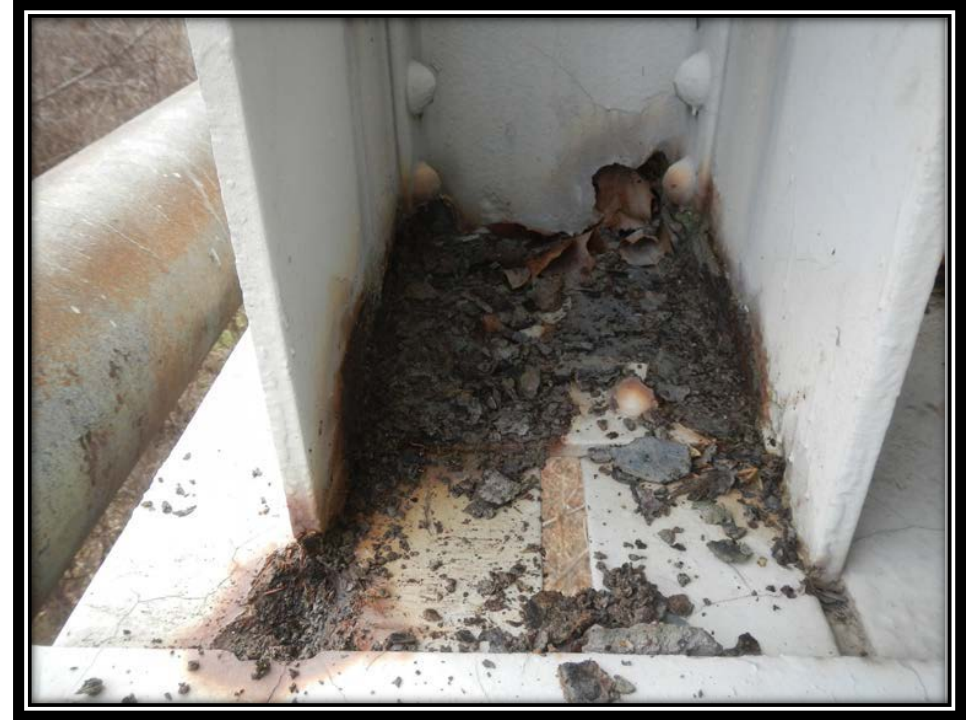
Looking west at L5L6 at L6, south truss in span 16. Note: 1/8-inch deep by 1-inch wide pitting on the top flange of the lower chord.
