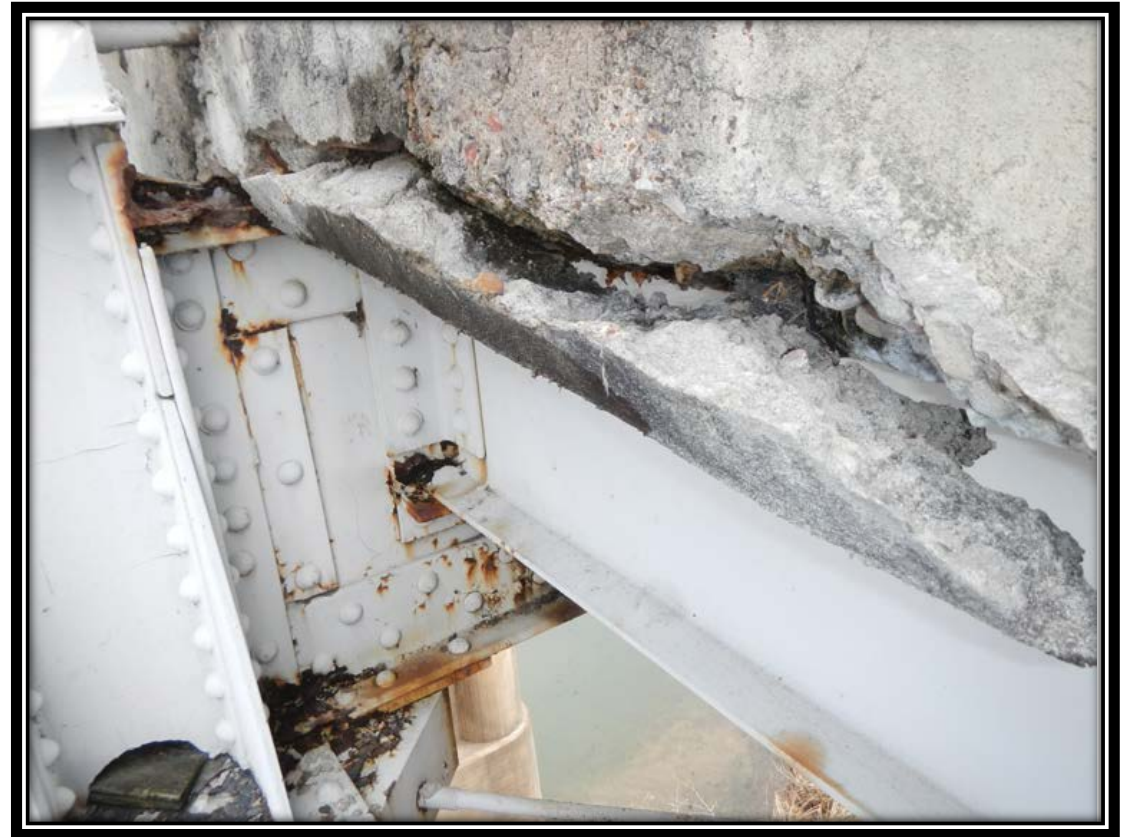
Looking southeast at the north edge of the deck at panel point 7 in span 16. Note: 3-foot long spall in the edge of the deck with exposed reinforcing steel.
