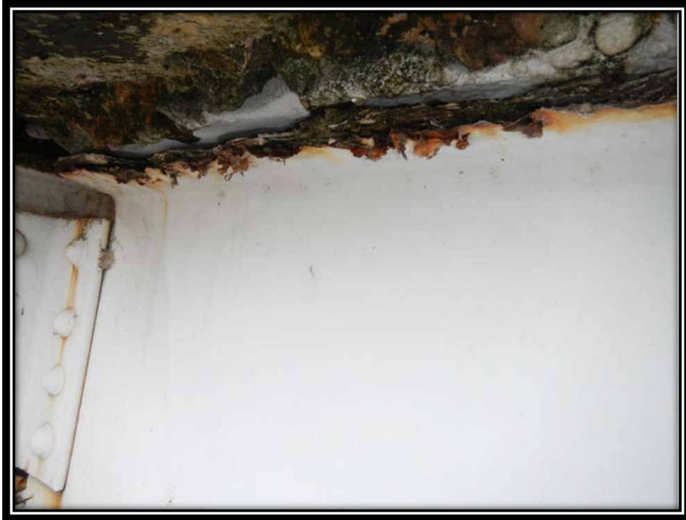
Looking southeast at stringer 1, span 16 at floor beam 7. Note: 1-inch wide knife edge section loss to the stringer top flange for 10-feet of stringer length.
