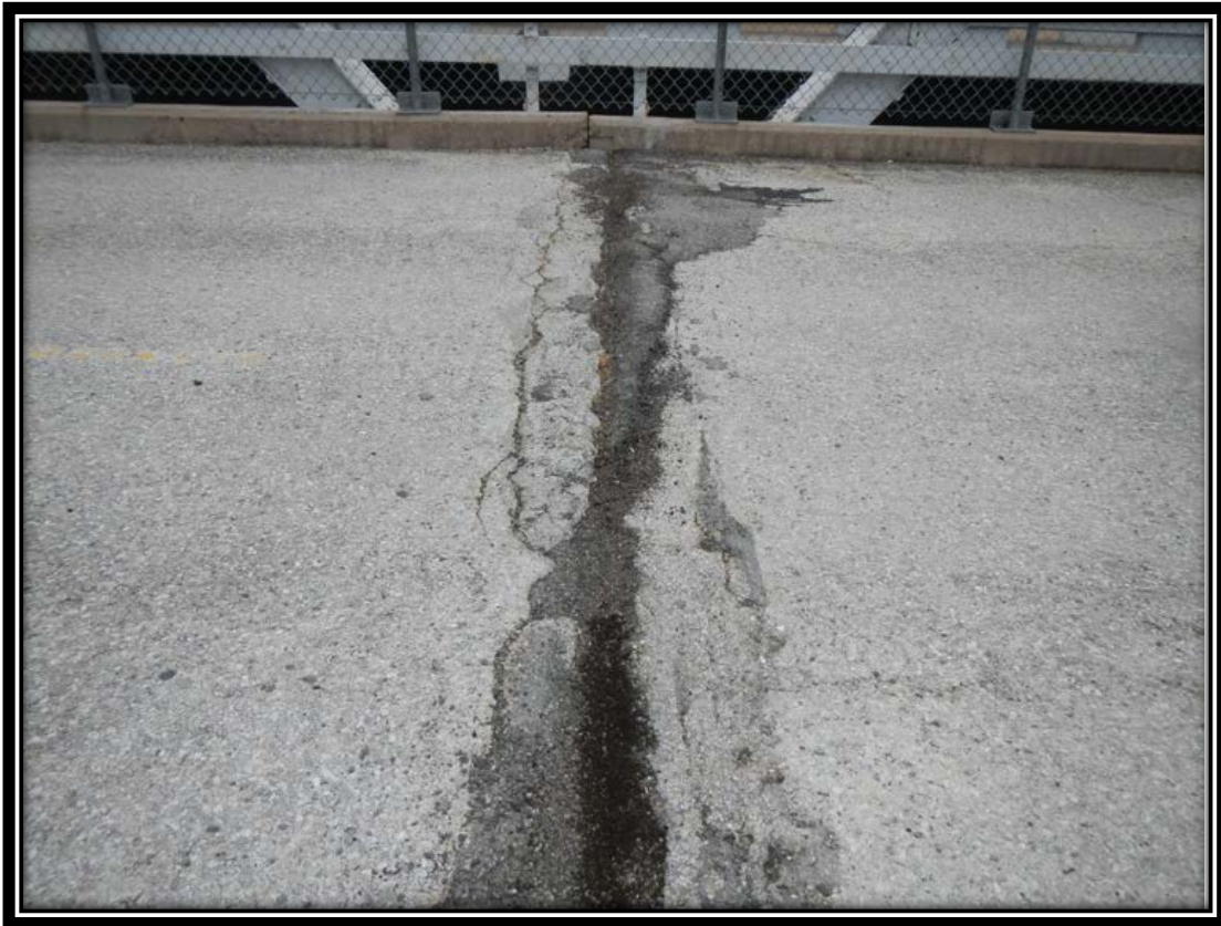
Looking north at the asphalt wearing surface over pier 17 between spans 17 and 18. Note: the asphalt patch is loose and deteriorated.
