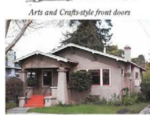
Short paired boxed columns on top of shingled, tapered pedestal
