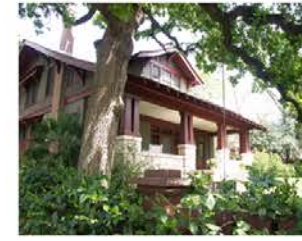
A shed-roof porch continues the line of the primary roof with a change in the slope
