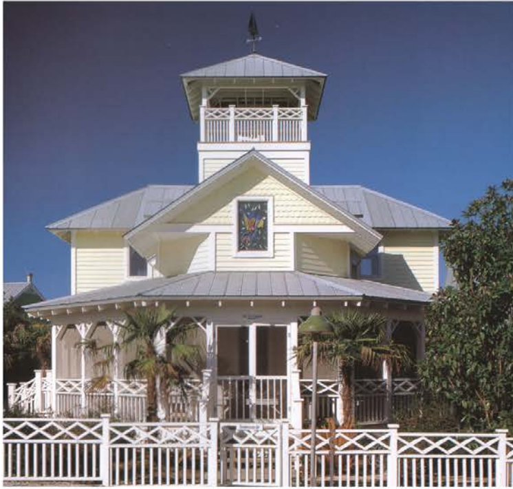
An example of tower design well coordinated with the rest of the house
