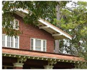
Picture window with flanking double-hungs with divided lites in upper sash
