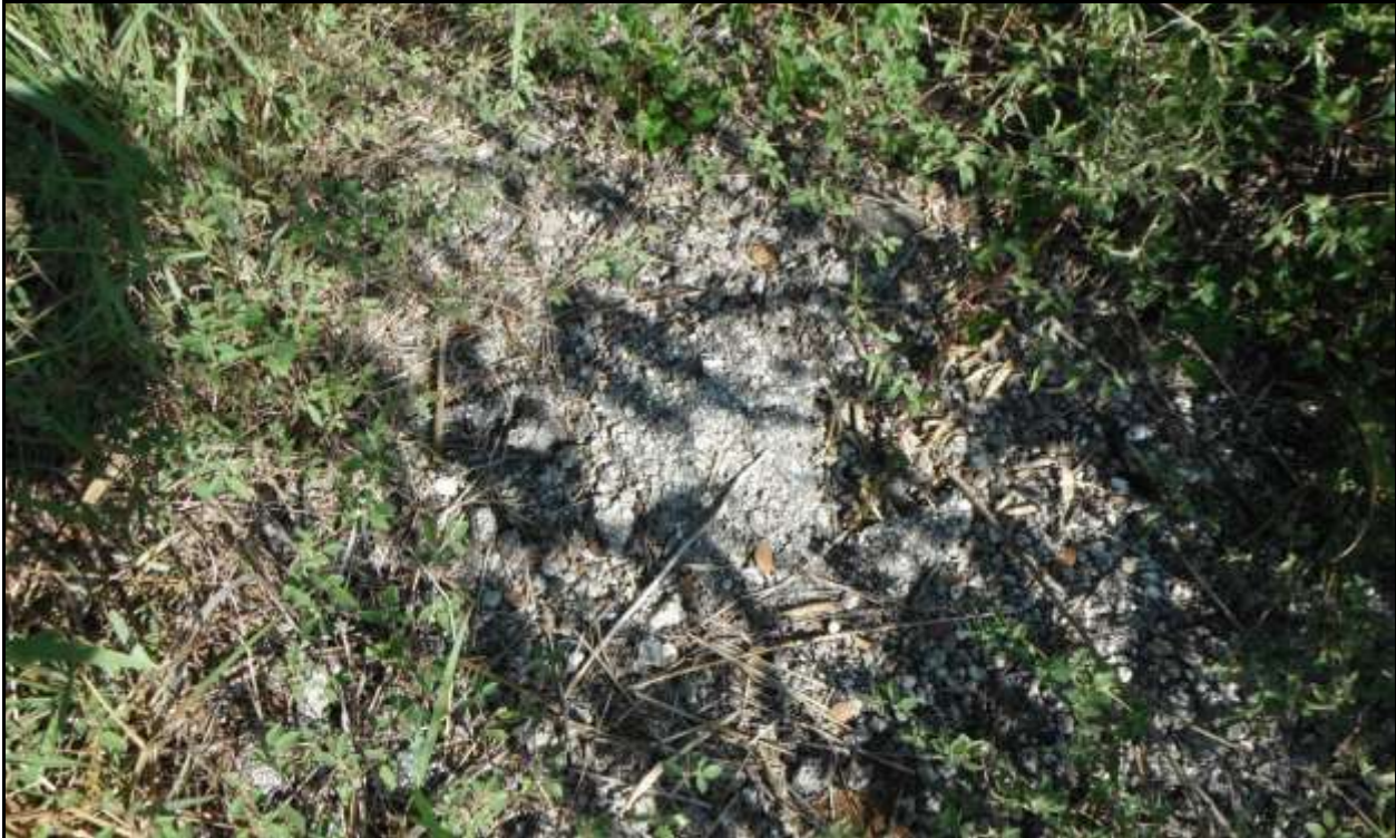
Figure 2-6. Asphalt west of tributary of Gills Branch within earlier alignment of SH 21
