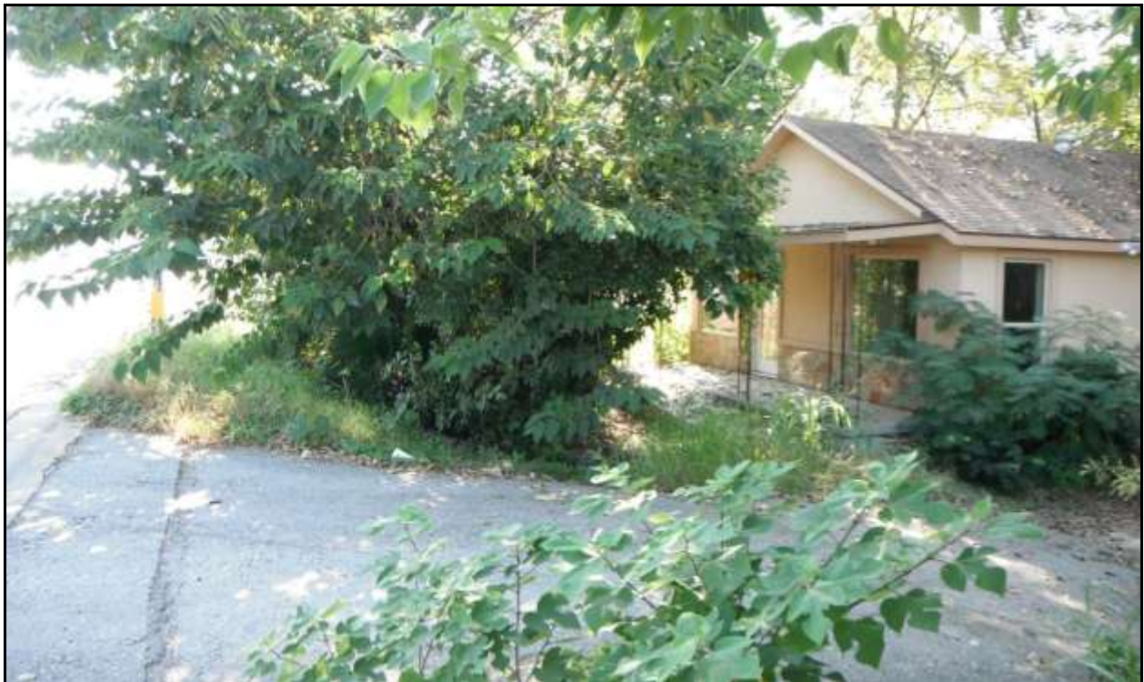
Figure 2-2. Modern structure near west end of Project Area, facing east
