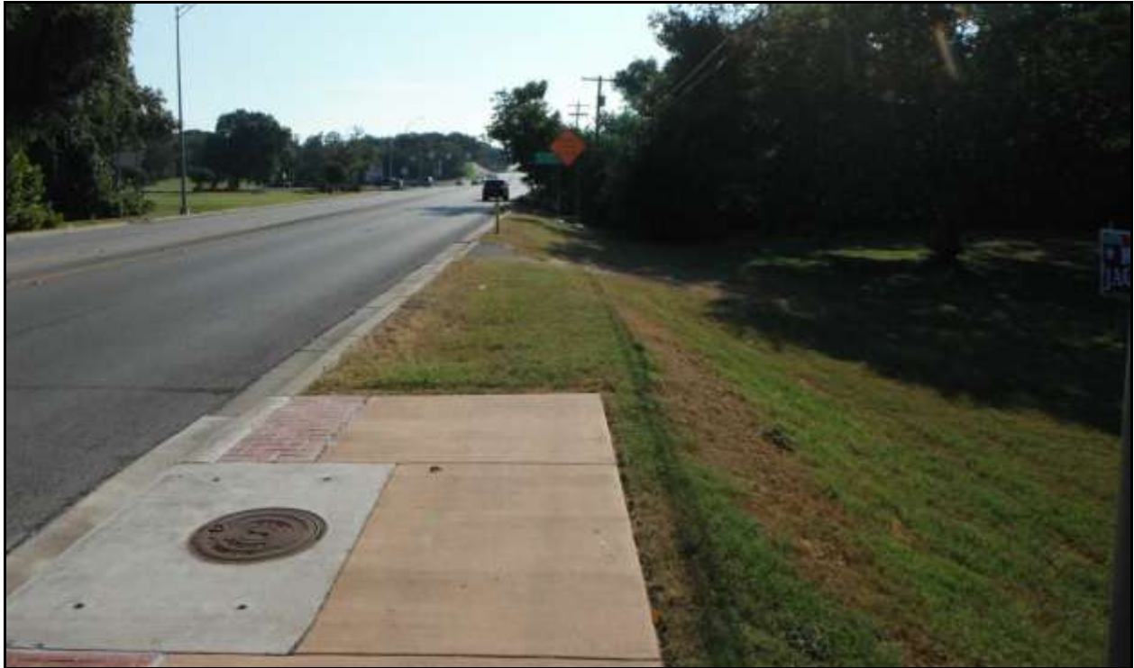
Figure 2-1. West end of Project Area on artificial berm, facing east
