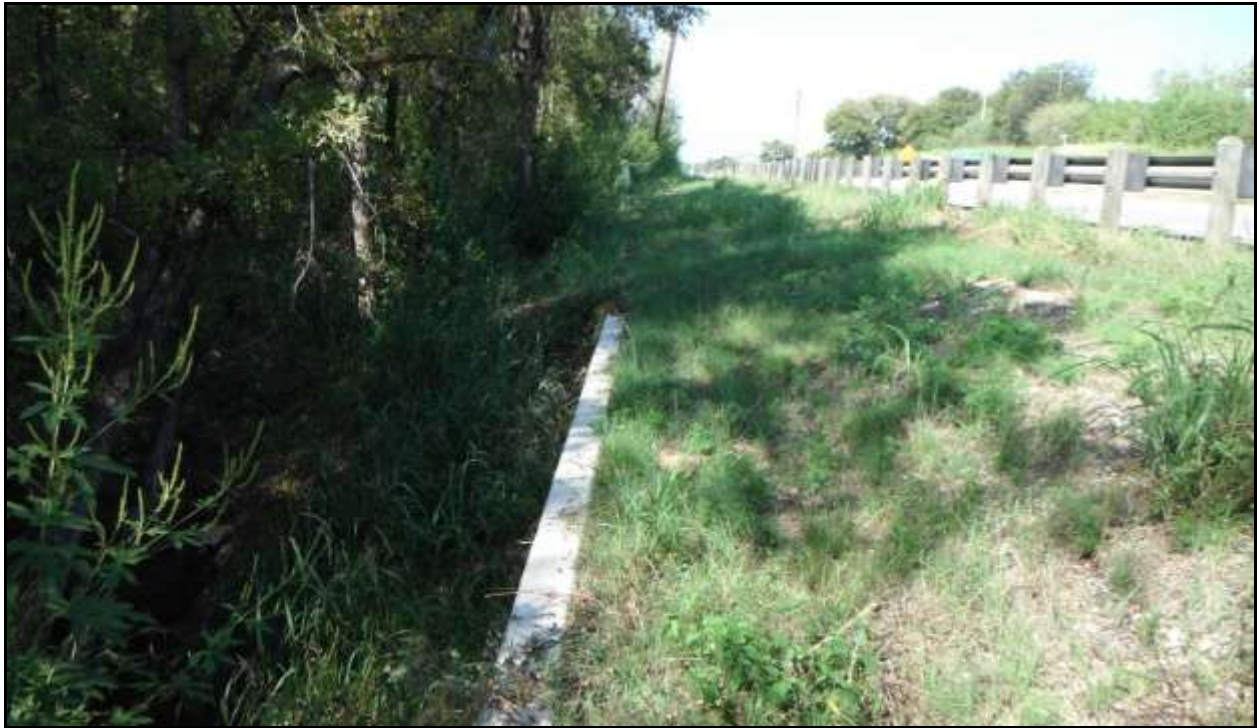
Figure 2-7. Artificial berm and bridge over tributary of Gills Branch, facing west
