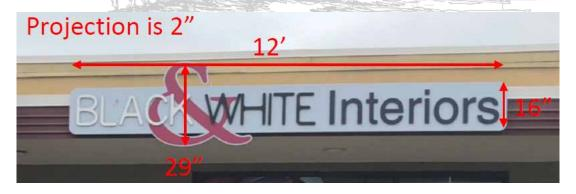
The sign will be mounted with L bracket to the wall face and project approximately 2 inches from the wall. No sign lighting will be added.
