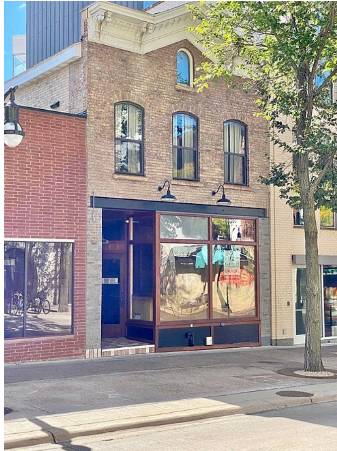
Figure 4-1 Original Cornice on Historic Masonry Building
