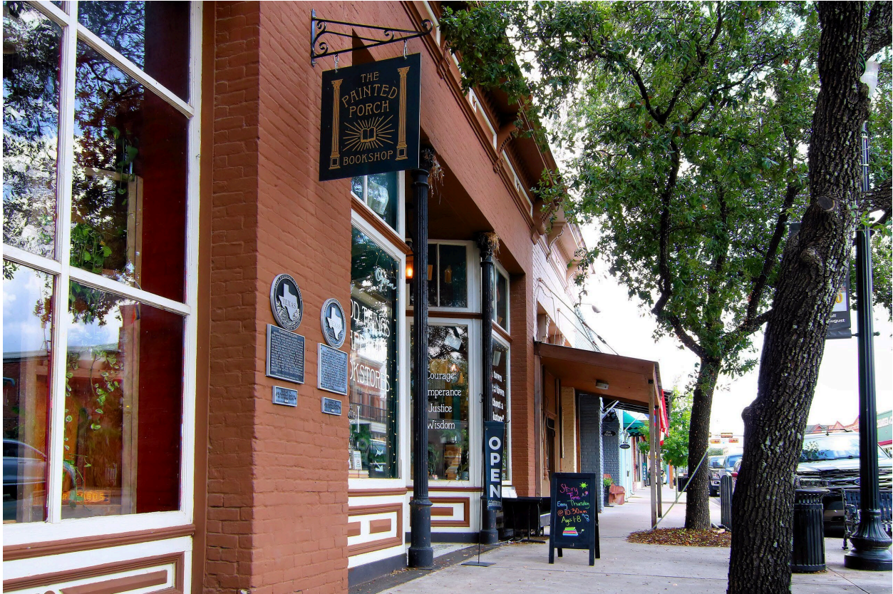
Figure 3-1 Downtown Historic District Streetscape
