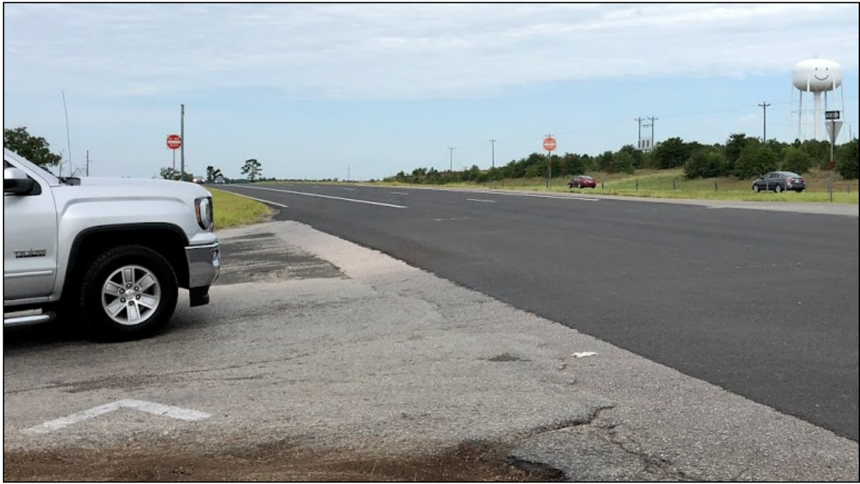
Figure 4. View looking left/west from NB McAllister Rd approach to SH 71 showing faded DO NOT ENTER signs, deceleration area striped into the previous 10' shoulder (leaving no shoulder), and sight distance limitation.
