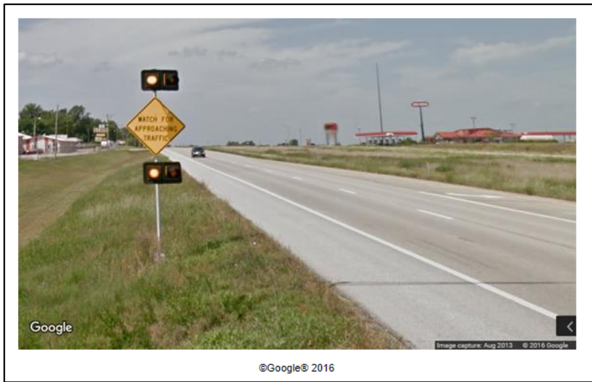
Figure 10: Example of an Intersection Conflict Warning System, Missouri (Source: Google Maps, 2016)
