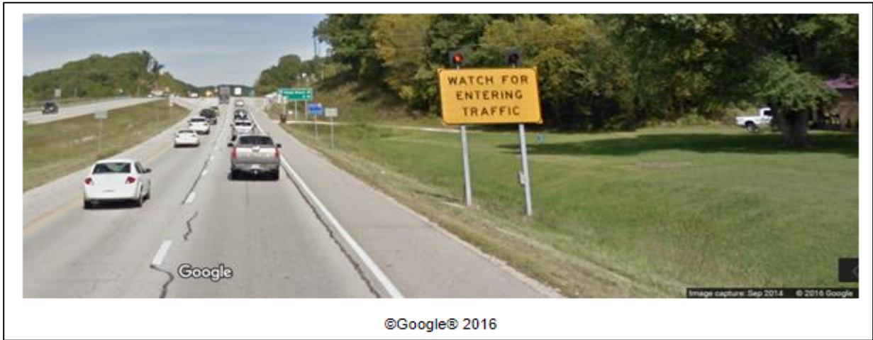
Figure 9: Example of ICWS installation of mainline signing, Missouri (Source: Google Maps, 2016)
