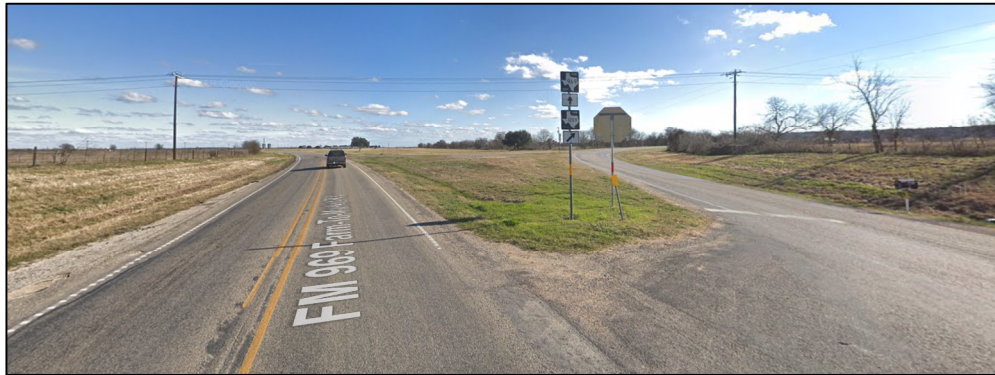
Figure 17: FM 1209 at FM 969 Northwest Leg, facing South (Google Maps, 2019)
