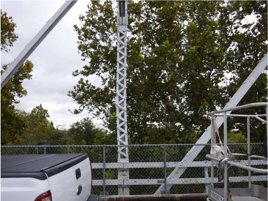
Photo 35 - Condition of Vertical Member L2U2, Truss 1, Span 6
