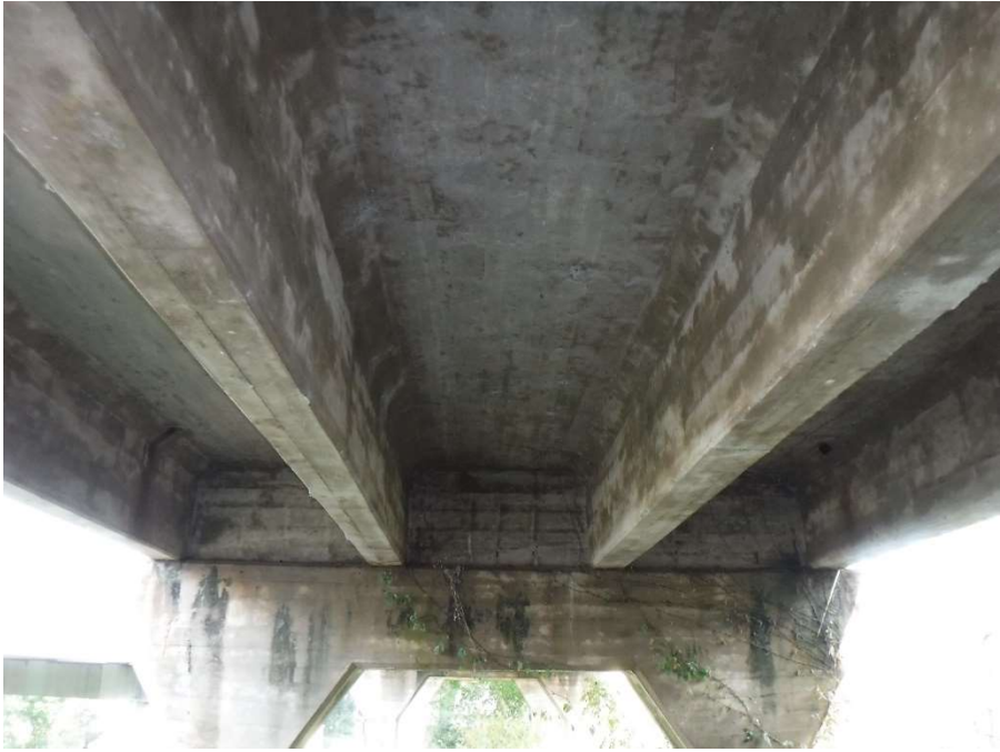
Photo 3 - Typical Approach Bridge Substructure
