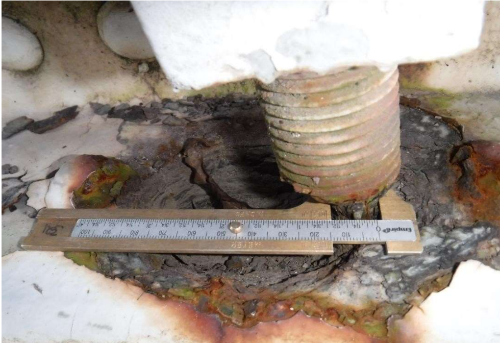
Photo 103 - Exterior anchor bolt condition at Joint L9, Truss 1, Span 5
