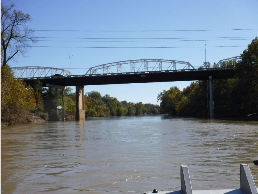
Photo 6 - Main Spans Looking Downstream
