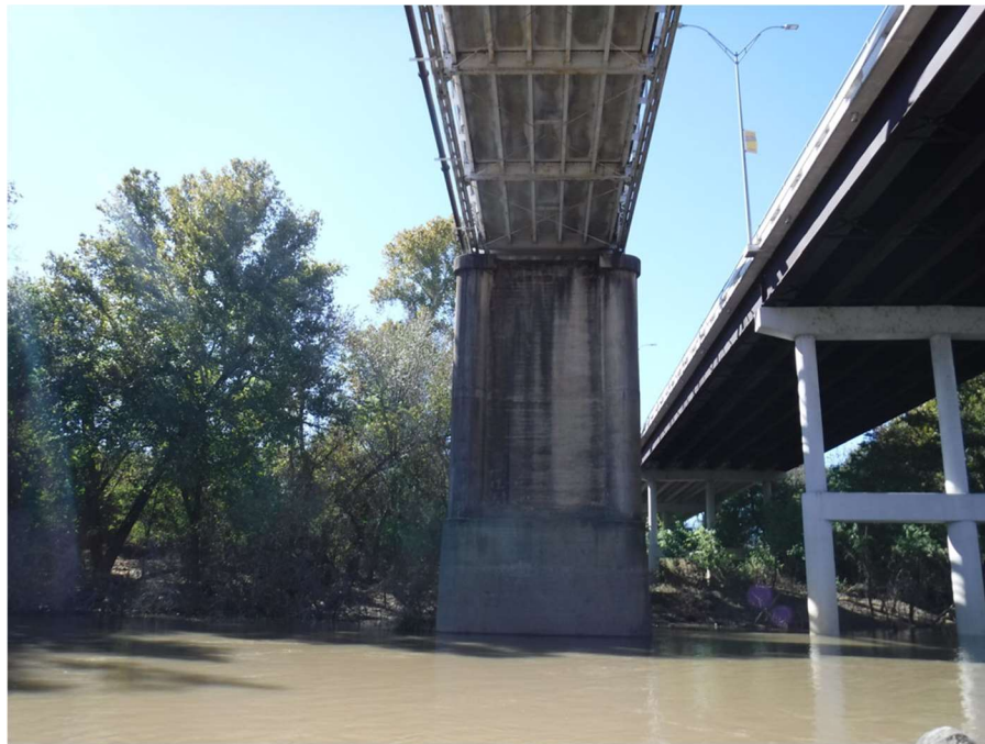
Photo 115 – Main substructure configuration, Bent 3
