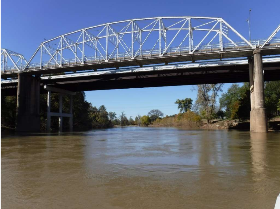
Photo 5 - Span 5 Looking Upstream
