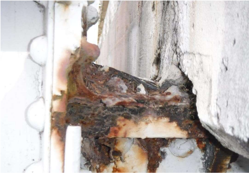
Photo 94 - Floorbeam to vertical connection angle condition at Joint L5, Truss 2, Span 6
