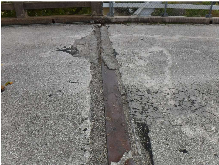
Photo 10 - Typical Joint at Approach Span and Main Span Interface
