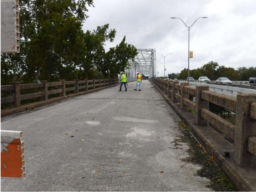
Photo 1 - East Approach Bridge Deck (Spans 1-3)
