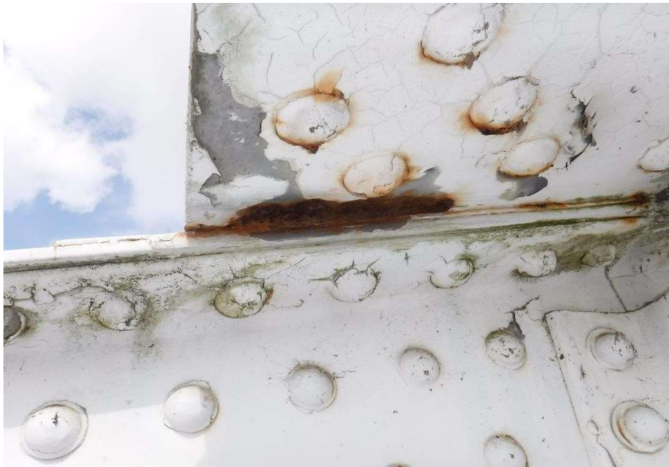
Photo 79 - Upper chord gusset plate condition at Joint U7, Truss 2, Span 4
