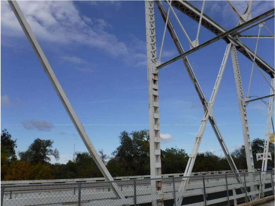
Photo 37 - Lower Half Replacement of Members L4U4 and L5U5 in Truss 2, Span 4
