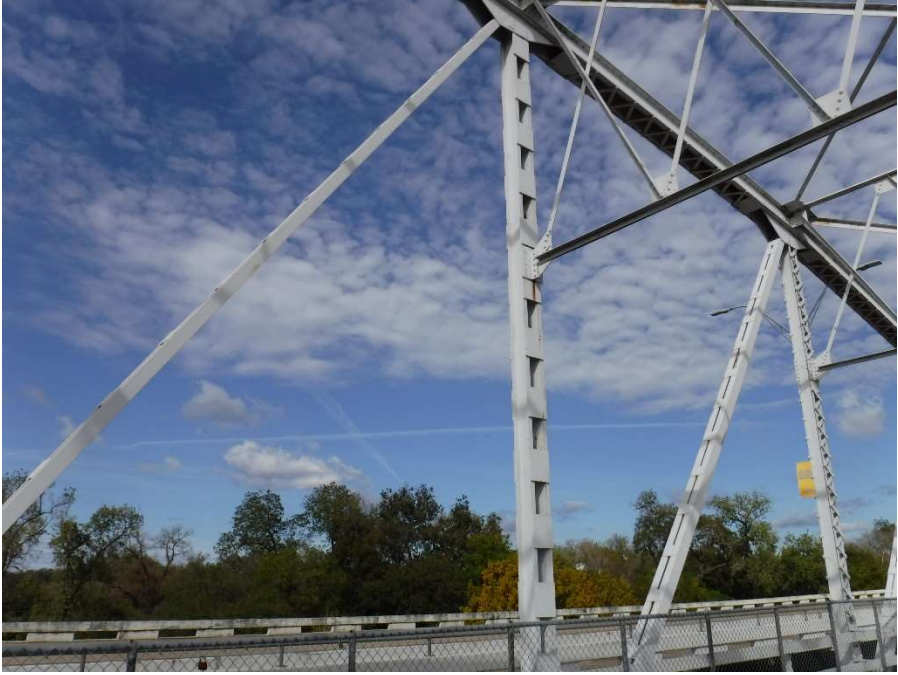
Photo 38 - Full Length Replacement of Member L6U6, Truss 2, Span 4
