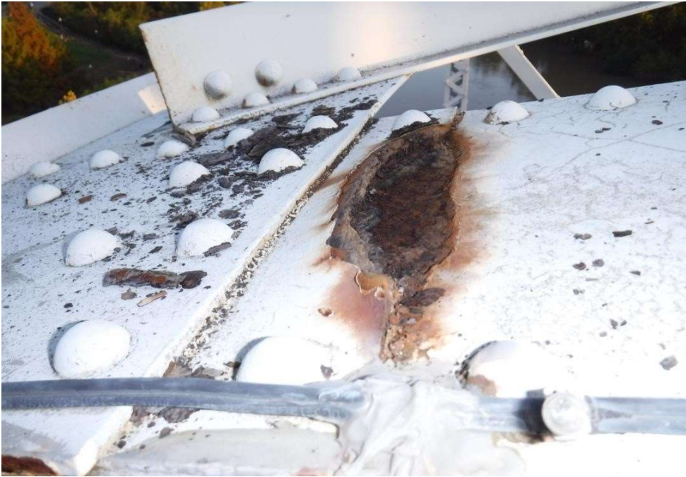
Photo 84 - Upper chord filler plate condition at Joint U1, Truss 2, Span 5
