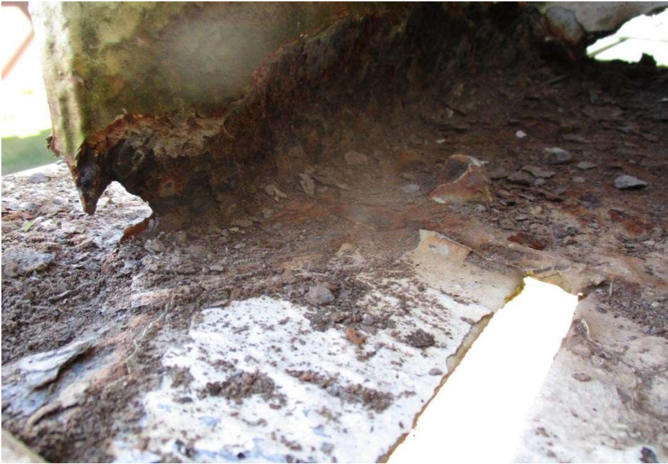
Photo 60 - Lower chord gusset plate condition at Joint L5, Truss 2, Span 4
