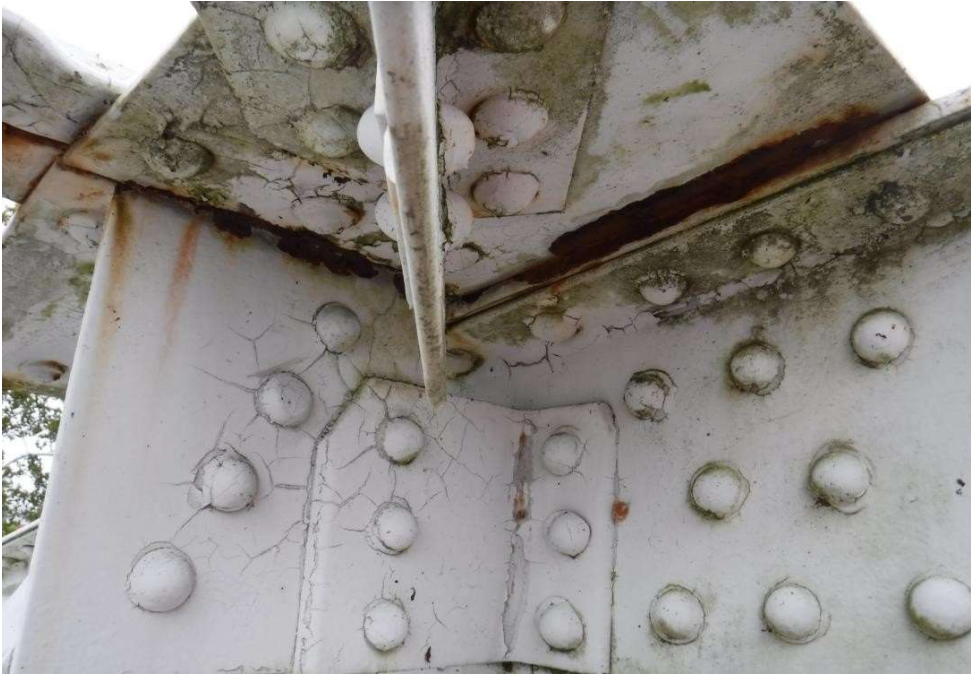
Photo 77 - Upper chord gusset plate condition at Joint U2, Truss 1, Span 4
