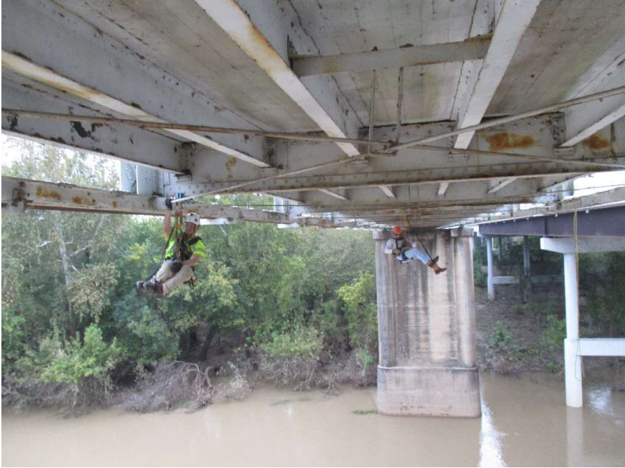
Photo 8 - Typical Floor System Layout
