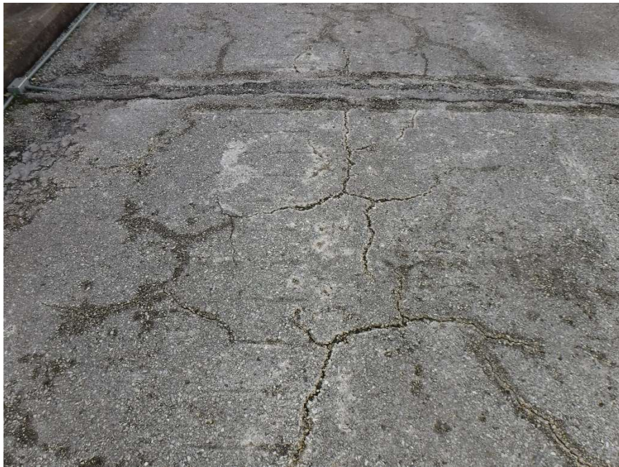
Photo 9 - Typical Approach Bridge Deck Joint
