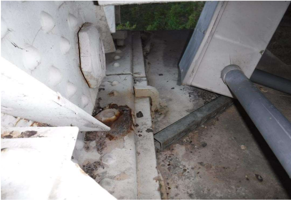
Photo 104 - Interior anchor bolt condition at Joint L9, Truss 1, Span 5
