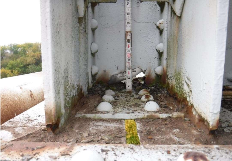
Photo 55 - Lower chord gusset plate condition at Joint L4, Truss 1, Span 4
