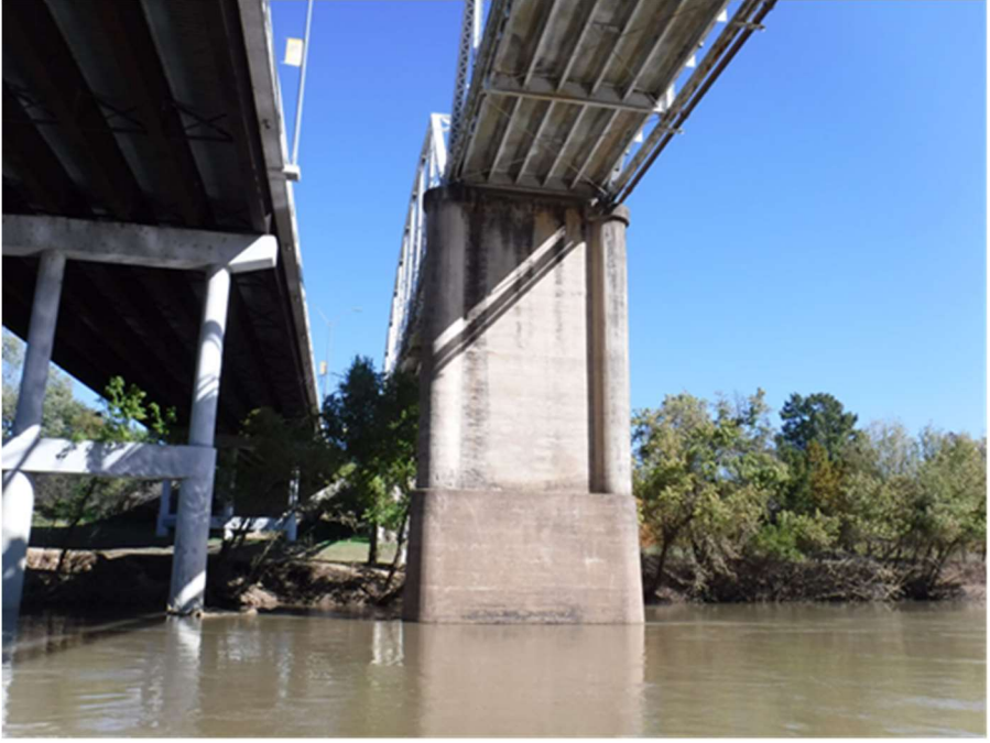
Photo 114 – Main substructure configuration, Bent 2
