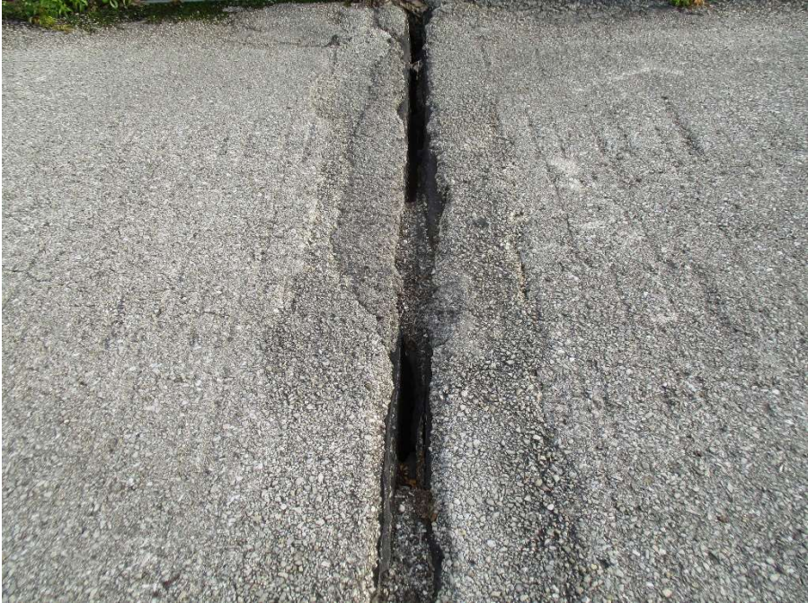
Photo 11 - Typical Deck Joint at Main Spans
