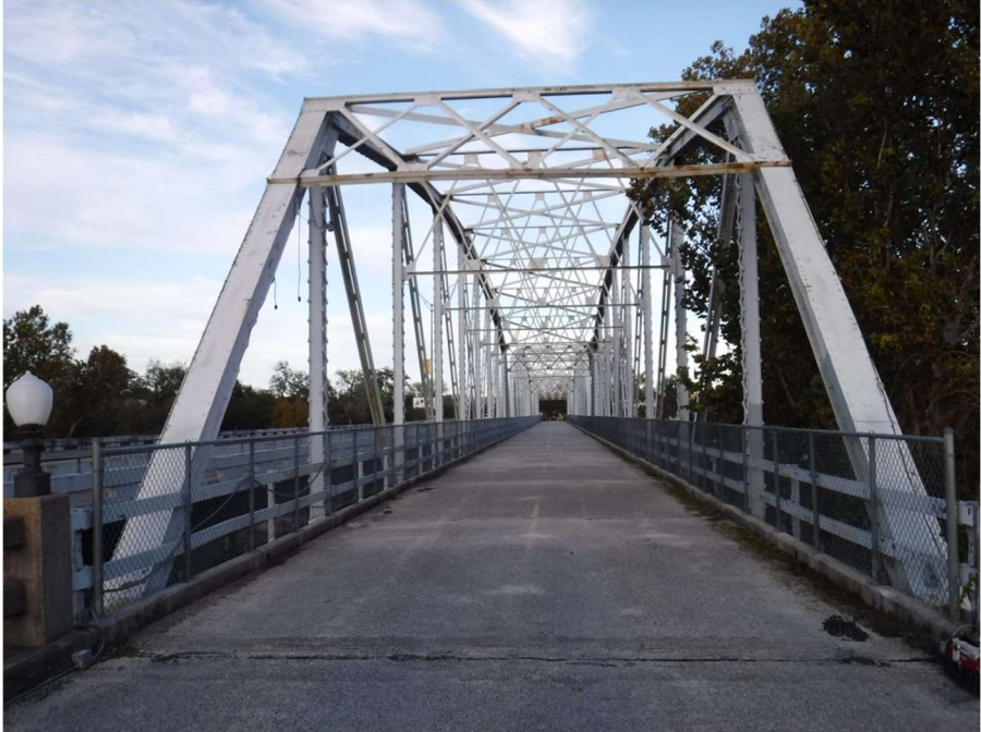
Photo 111 – Roadway over bridge
