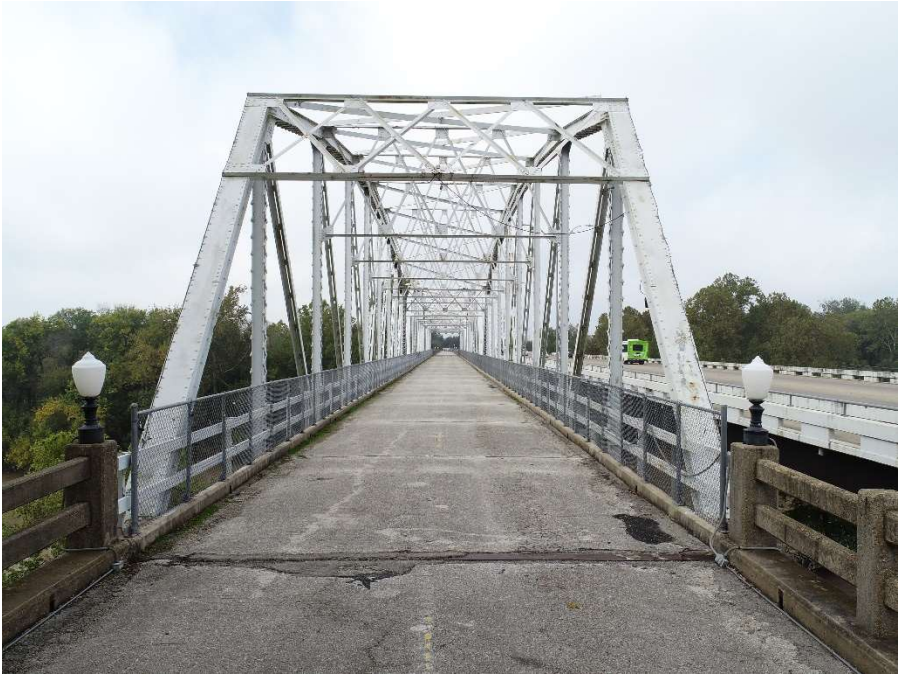
Photo 7 - Typical Parker Truss Cross Frames
