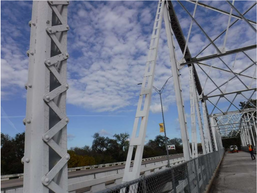
Photo 41 - Full Length Replacement of Diagonal Members L5U6 and L6U7, Truss 2, Span 5
