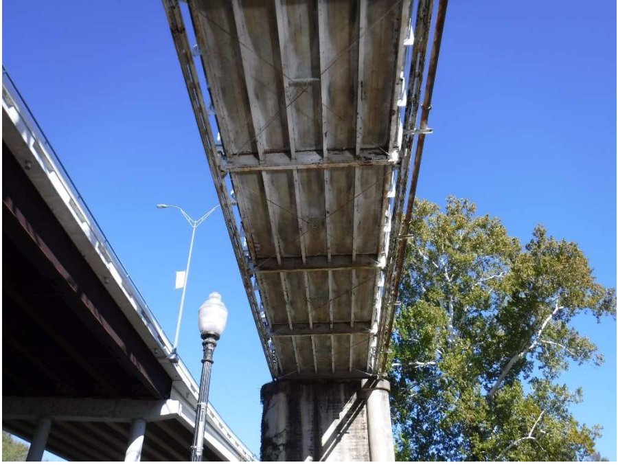
Photo 4 - Typical Main Span Substructure
