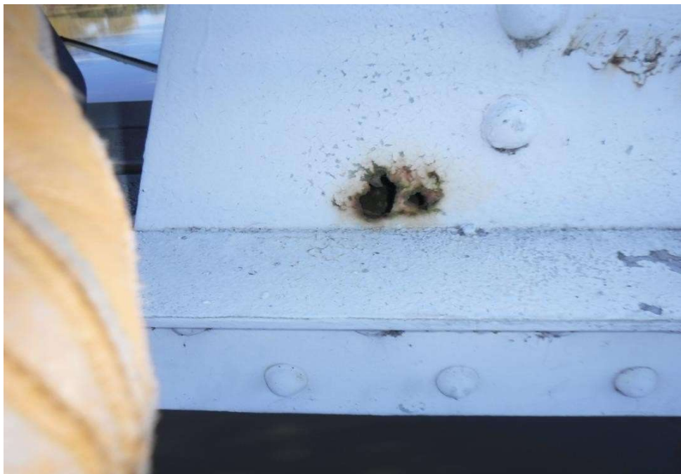
Photo 66 - Lower chord gusset plate condition at Joint L6, Truss 2, Span 5
