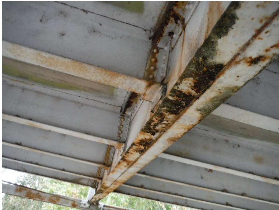
Photo 47 - Typical Interior Floorbeam Condition
