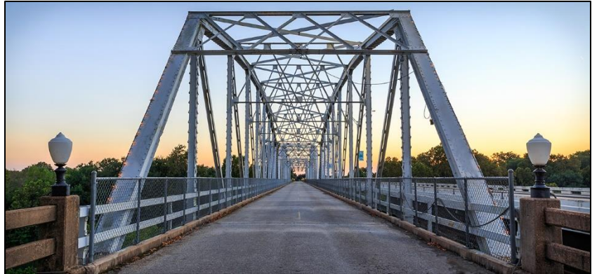
Figure 1: Old Iron Bridge
