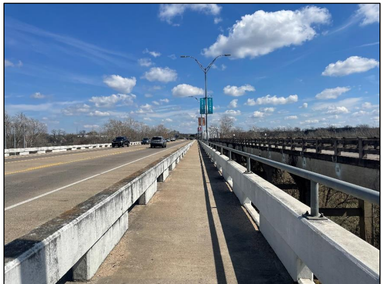
Figure 4: Existing Sidewalk Adjacent to SL-150
