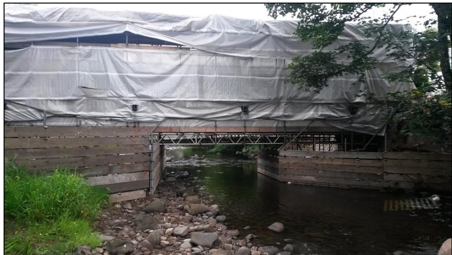
Figure 17: Example of Shrouded Lead Paint Removal Process
