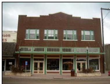
Addressing deteriorating elements in historic buildings (transom windows, storefront) and aesthetics (cleaning, paint) can give an already green building new life as this recent project in Hillsboro shows. (top to bottom: existing, TMSP rendering, and completed project.)
