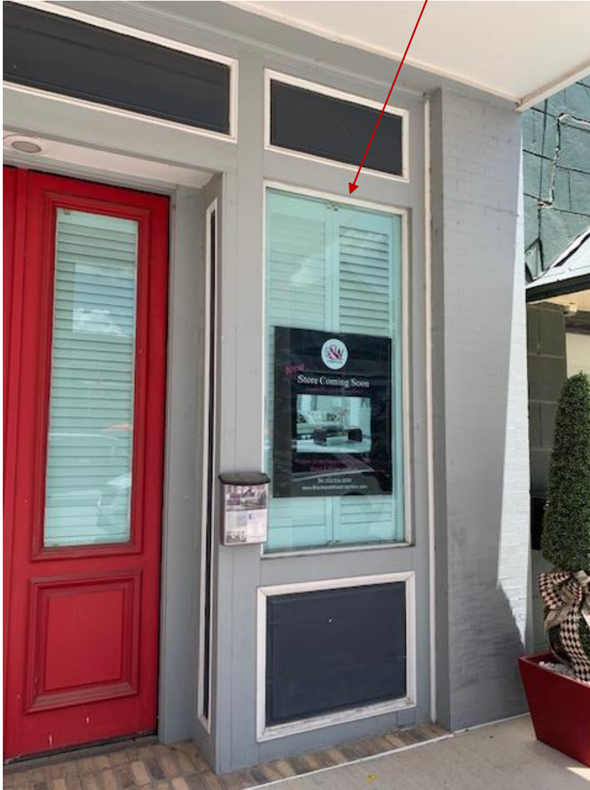
Present Window Front on Right Side
