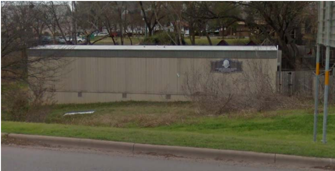
Existing Temporary Building
