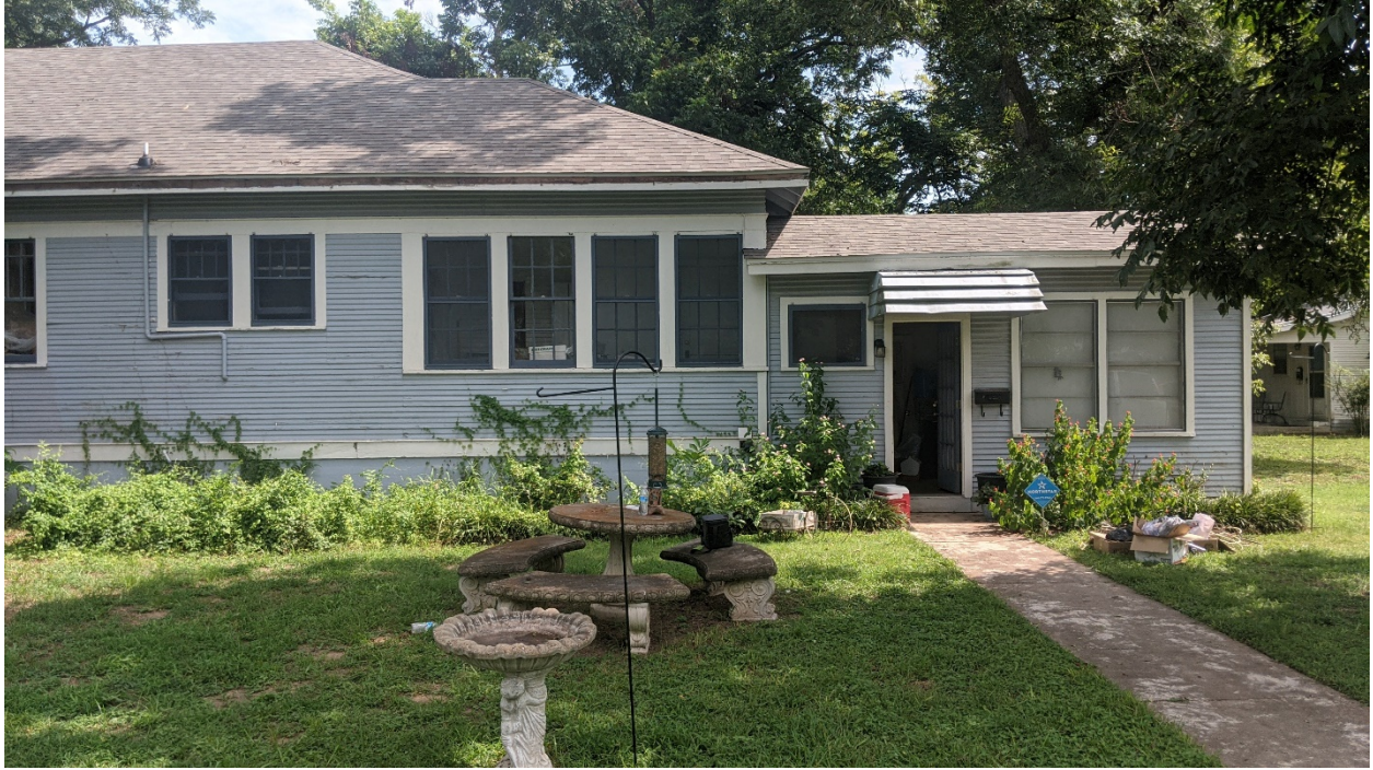
Figure 5 North Side from Elm St
