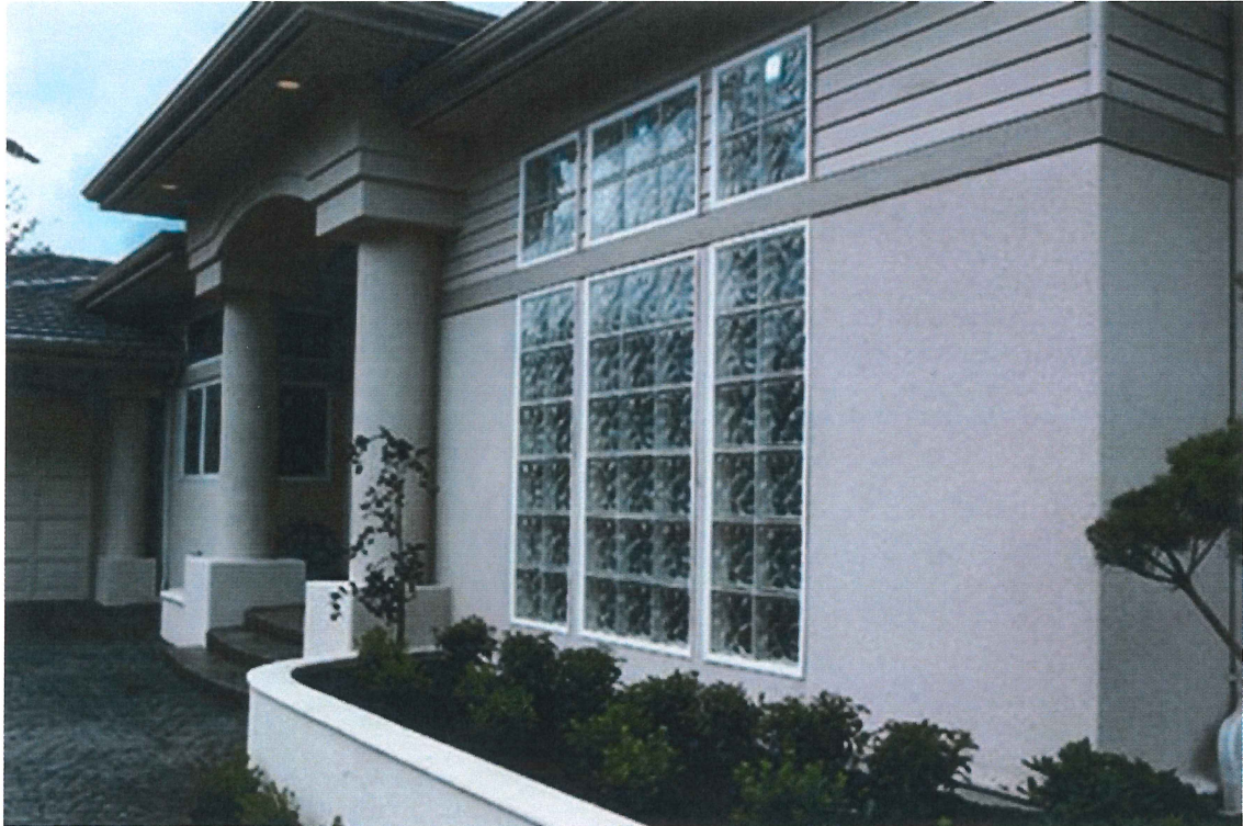
3. Metal Exterior Construction
